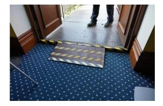
and the portable ramp at the entrance to the threshold
