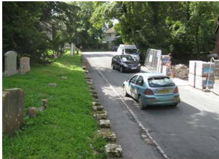
Church Hill, looking towards the blind bend outside St Mary's Church.
