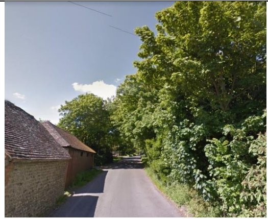
20. Firle Road looking north
