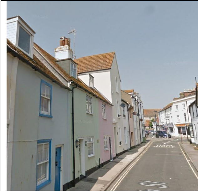
7. View northwards up Church Street towards the church
