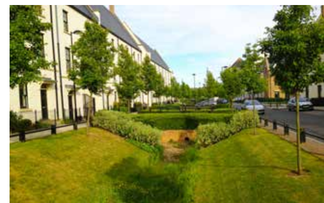
Figure 6: Example of a sustainable drainage system in Upton creating a public space whilst also providing flood alleviation.
