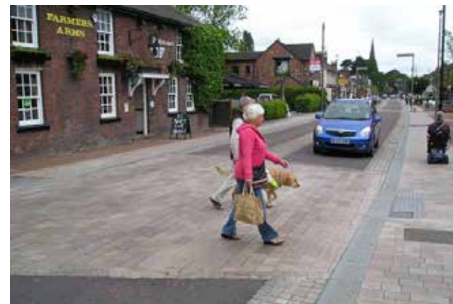
Figure 5: Positive example of a street in Poynton, Cheshire where the use of materials and vertical deflection, provide a pedestrian priority environment and is aesthetically pleasing.
