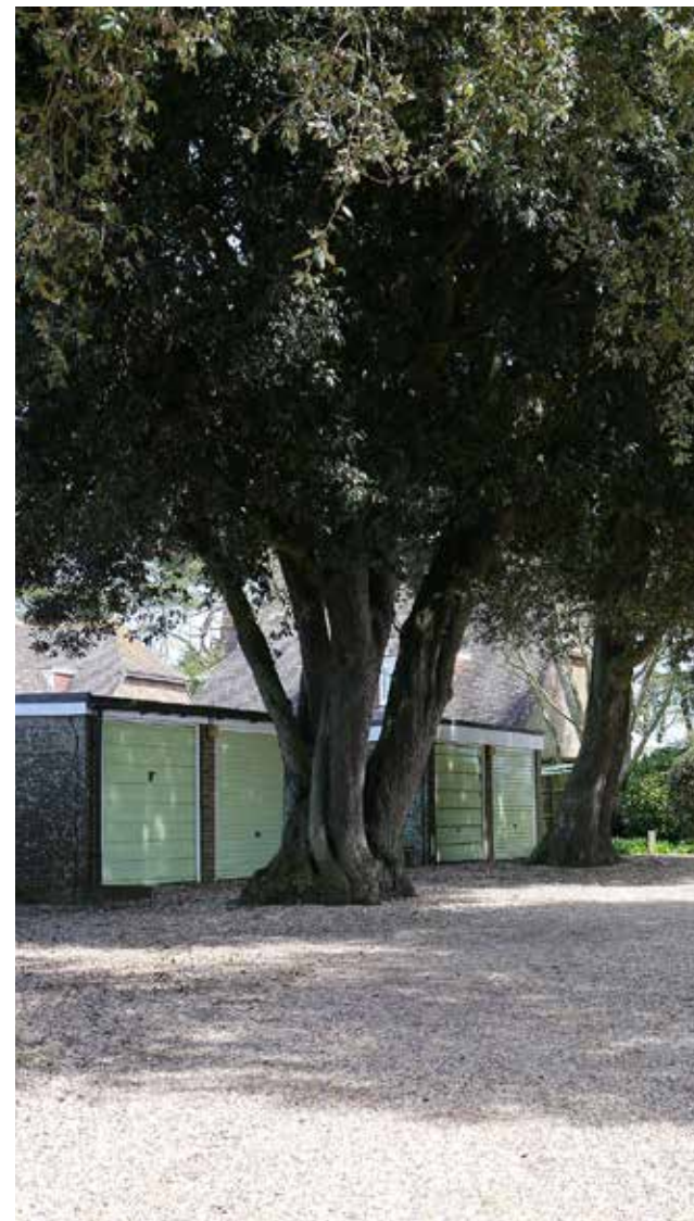
Figure 19: Example of tree that has grown too close to buildings and thus has created a potential conflict with circulation.
