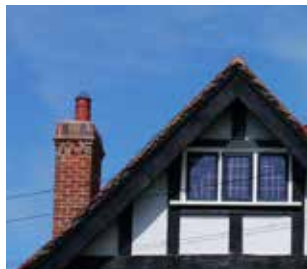
Gable ended roof
