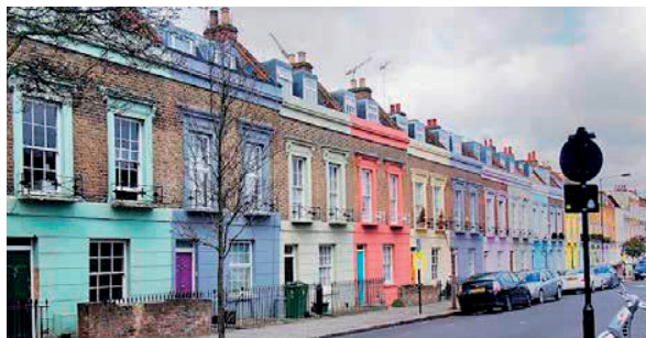
Coloured walls to improve the façade
