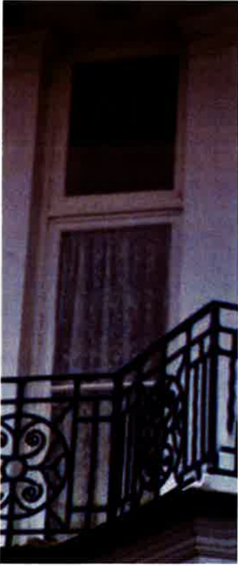
4. Timber framed sash window
