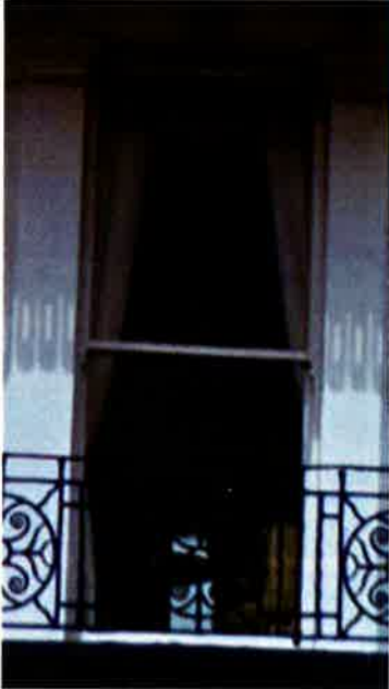
5. Timber framed sliding sash window
