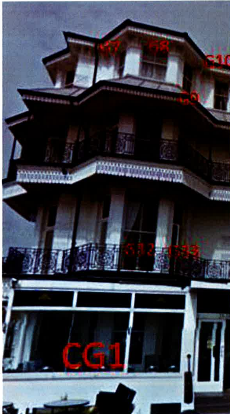
Photograph 9: Prior to works photos of South elevation facing Royal Parade (1)
