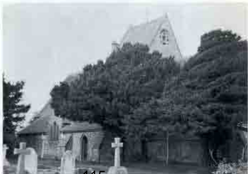
St. Mary's Church, North Common
