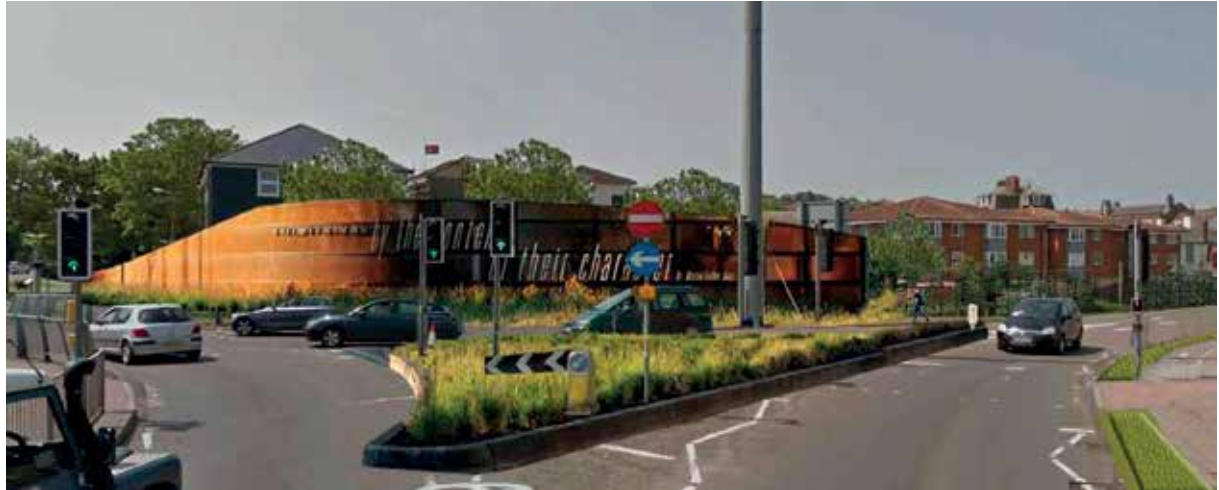
Figure 1 – Approaching the ring road from the swing bridge
