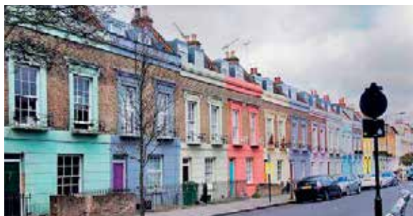
Coloured walls to improve the façade
