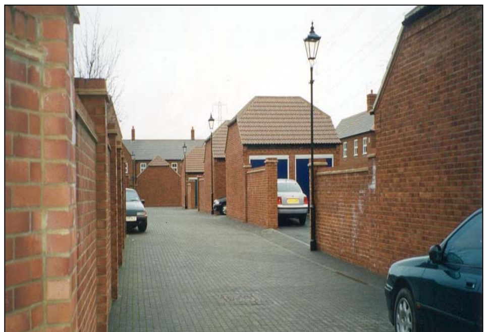
Visibility into and out of the parking bays is very poor creating hidden areas not observed by the surrounding development.
