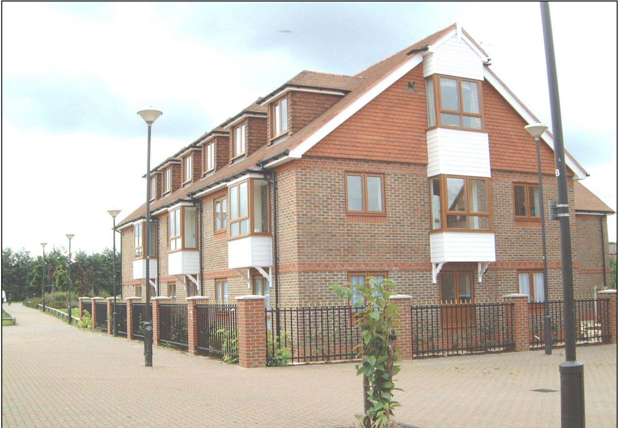
Development showing good boundary treatment, visibility and lighting.
