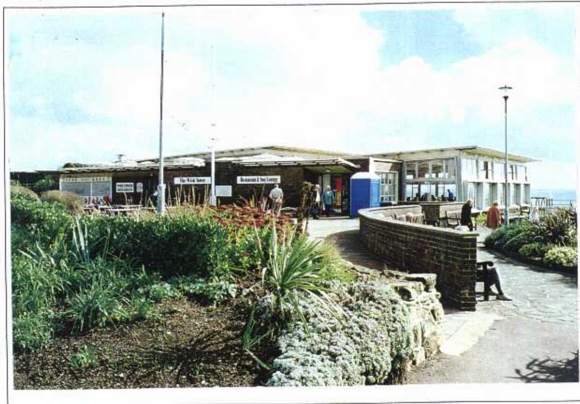
VIEW OF ENTRANCE FROM WEST
