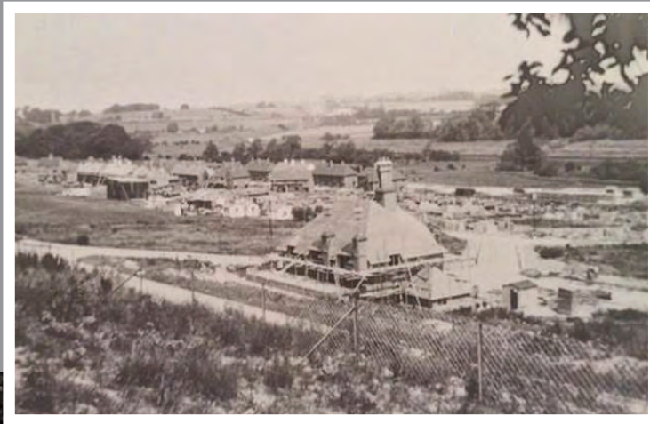
Landport Estate being built -1937
