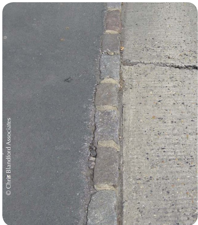
Granite block paving to demarcate crossing points in Peacehaven
