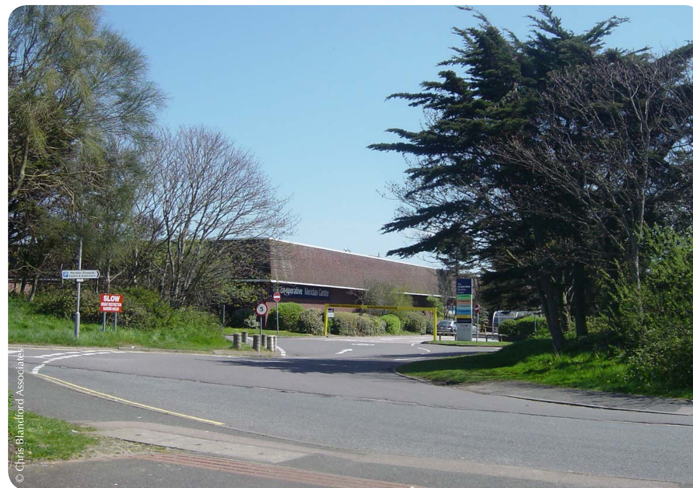
The Meridian Shopping Centre obscured by mature trees and landform with poor connectivity to surrounding areas
