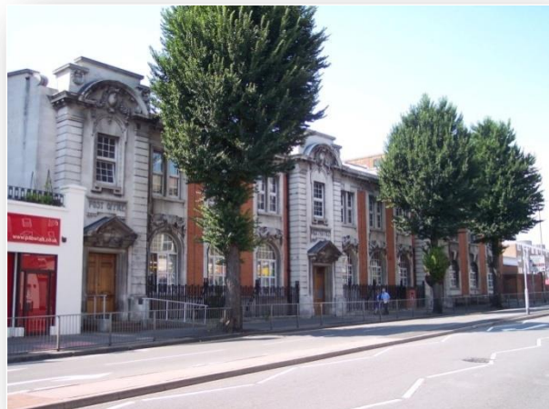
Picture 6 - Town Centre Development Opportunity Site 3
