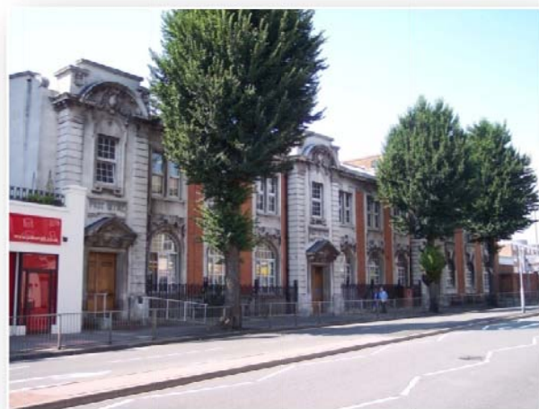
Picture 6 - Town Centre Development Opportunity Site 3
