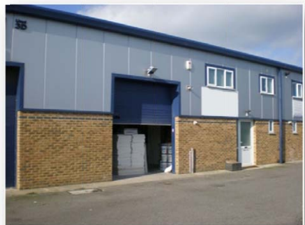
Picture 3 - Small units at Southbourne Business Park, Courtlands Road
