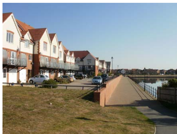
Figure 2 Housing at Brisbane Quay
