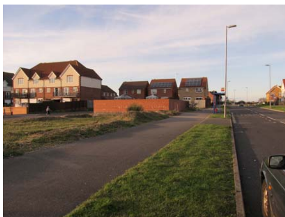
Figure 31 Pumping Station on Site 8
