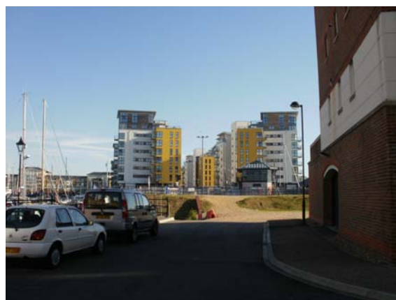
Figure 43 Land adjacent to the Lock Gates viewed from Key West
