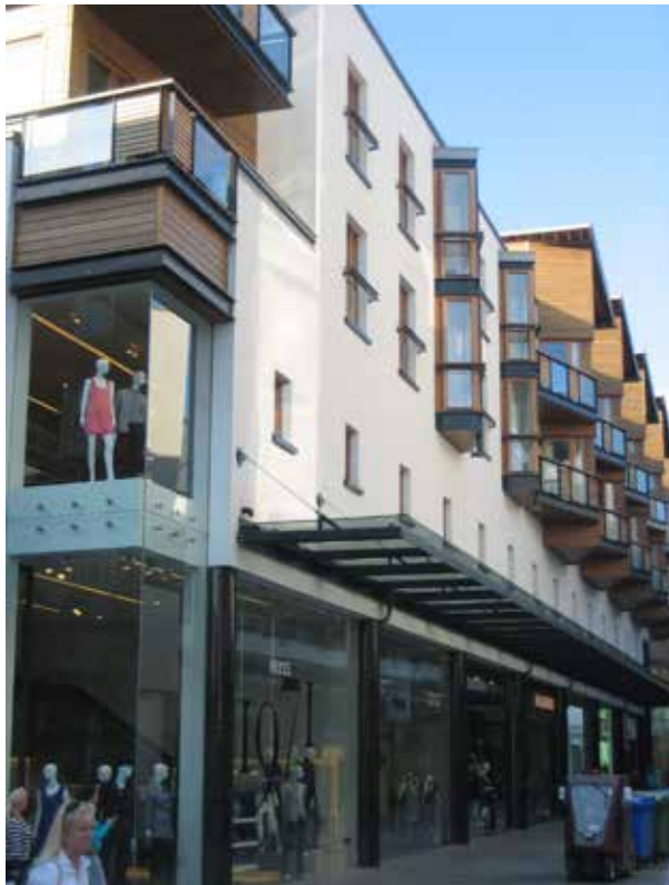
Different uses and building elements clearly expressed
