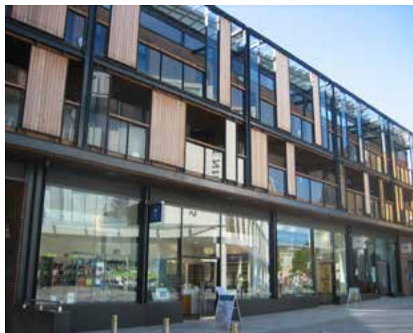
High quality mixed use development with apartments above retail
