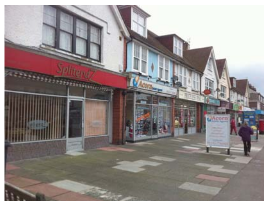
Seaside Local Shopping Centre
