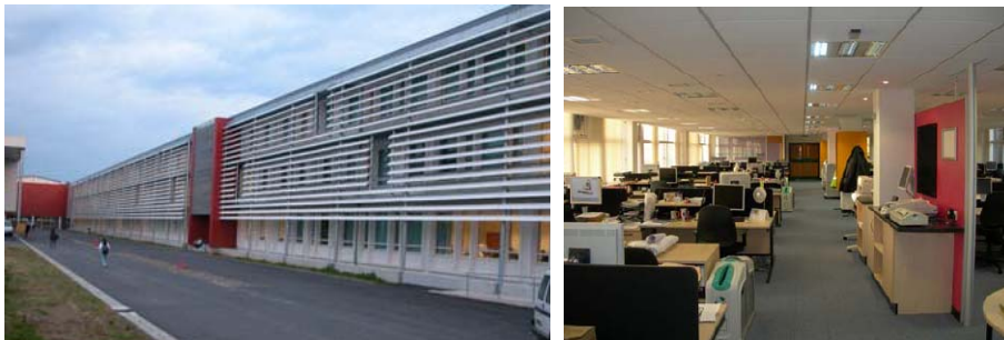
Figure 13 Strategies to improve energy efficiency in non-domestic buildings. Shading devices fitted to Lycée Chevrollier, a high school in France (left) and office layout of Stevenage Council offices after Accommodation Review. The existing cellular offices were converted into modern IT based 'open plan' office areas, with new modular desks and high efficiency layouts to improve occupancy levels. The number of unoccupied desks was reduced, and CRTs were replaced with pole mounted, flat screen computer monitors to reduce the desk area used by each employee. (right). (Source: REVIVAL project, AECOM) 17
