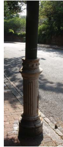
Picture 32 Vent pipe, Paradise Drive.
