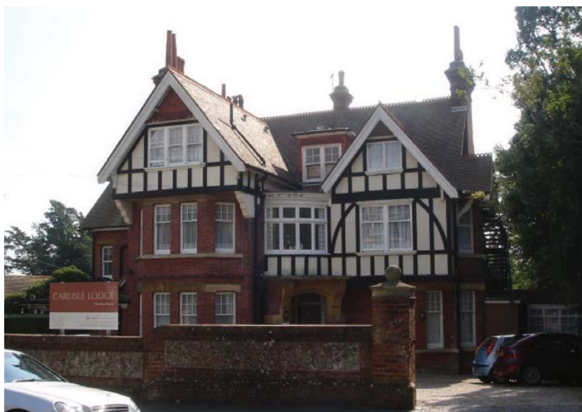
Picture 21 Property to Carlisle Road.
