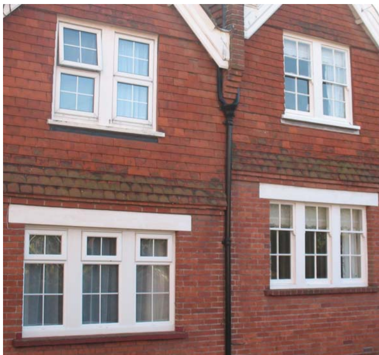
Picture 93 The Village, uPVC windows (left) and timber sash windows (right).
