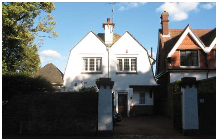
Picture 62 Darley Road, 1930s housing.
