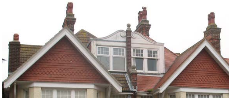
Picture 92 Concrete tiles & UPVC windows (left), clay tiles & timber sash (right).
