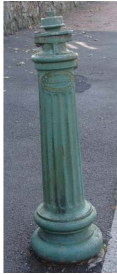
Picture 31 Water vent, Gaudick Road.
