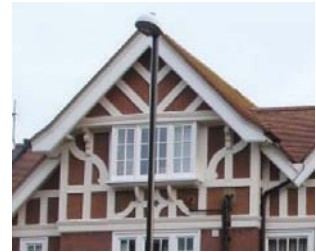
Picture 4 Timber detail to gable.
