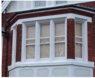
Picture 2 Timber sash windows.
