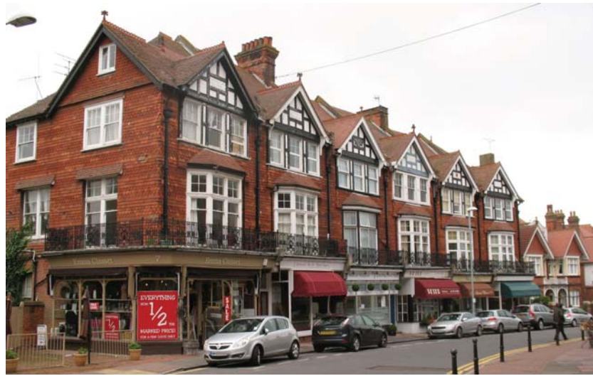
Picture 54 Meads Street nos. 7 - 17.
