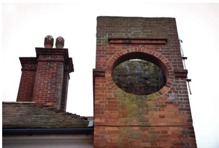
Picture 57 Detail of brick drill tower.
