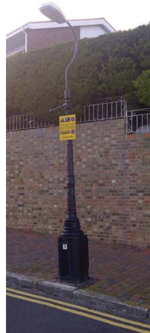
Picture 28 Square based gas lamp, South Cliff
