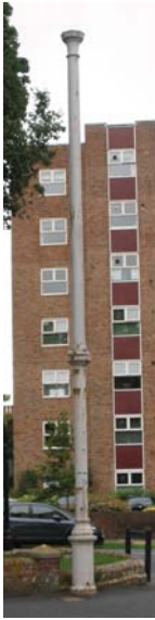
Picture 30 Vent pipe, Meads Road.
