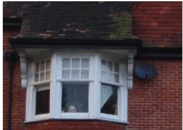
Picture 95 Satellite on front elevation.
