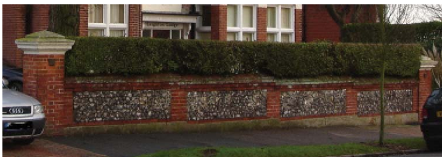
Picture 97 Brick & flint boundary wall.
