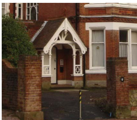
Picture 71 Decorative timber porch, Bolsover Rd.
