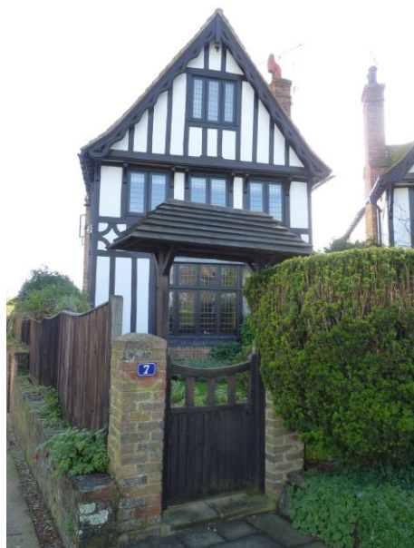
Left: installation of new gates to original gate piers.
