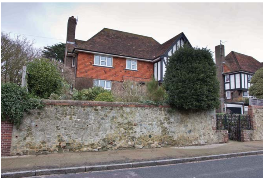
Picture 14 No. 3 Torfield Road, clay tile hangings and timber frame to gable.
