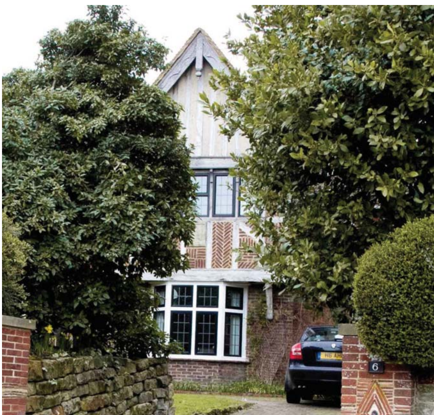
Picture 15 Decoative bargeboards and jetty to no. 6, Linston.
