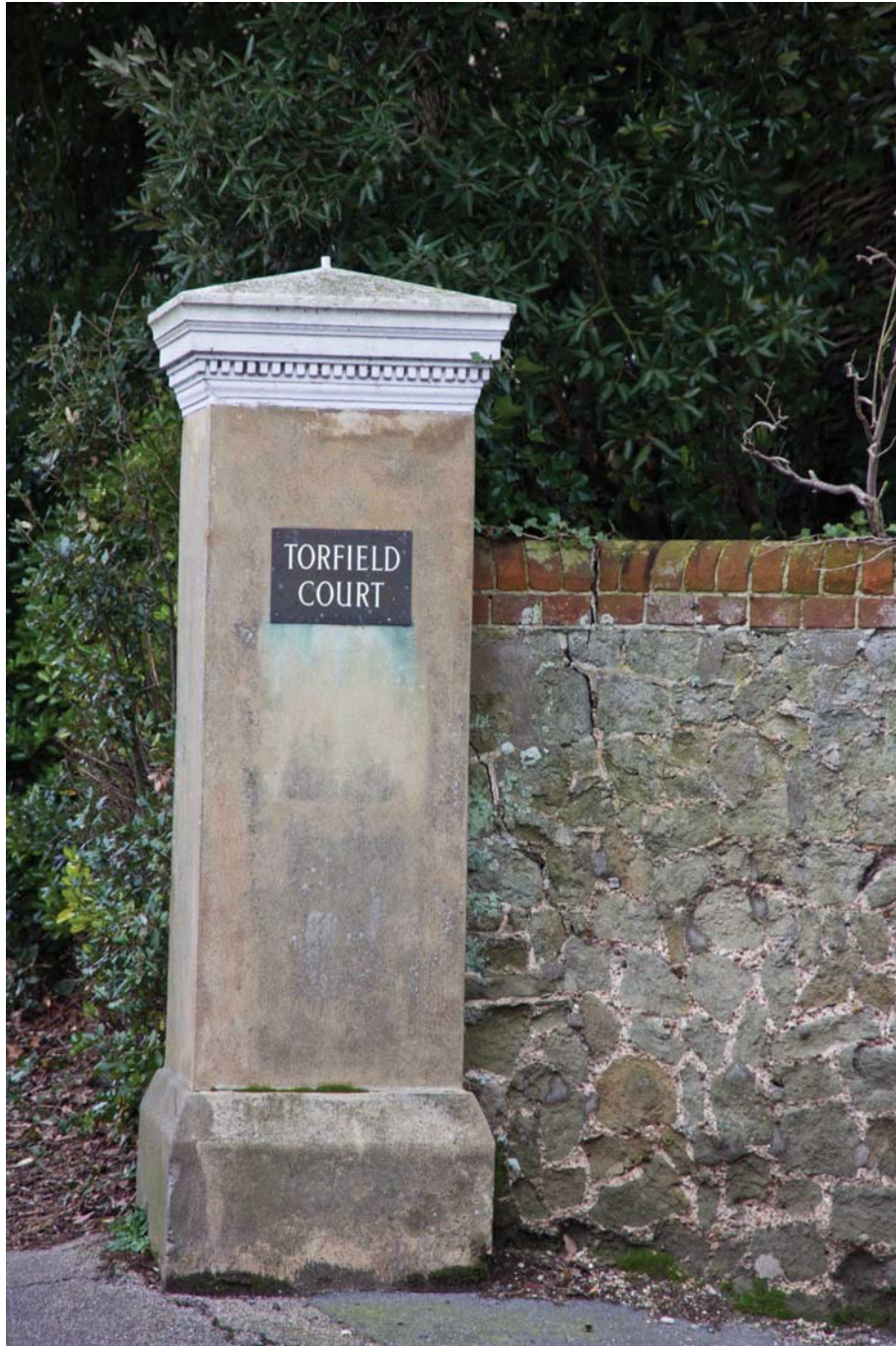
Picture 5 Torfield Court pier, St Anne's Road.
