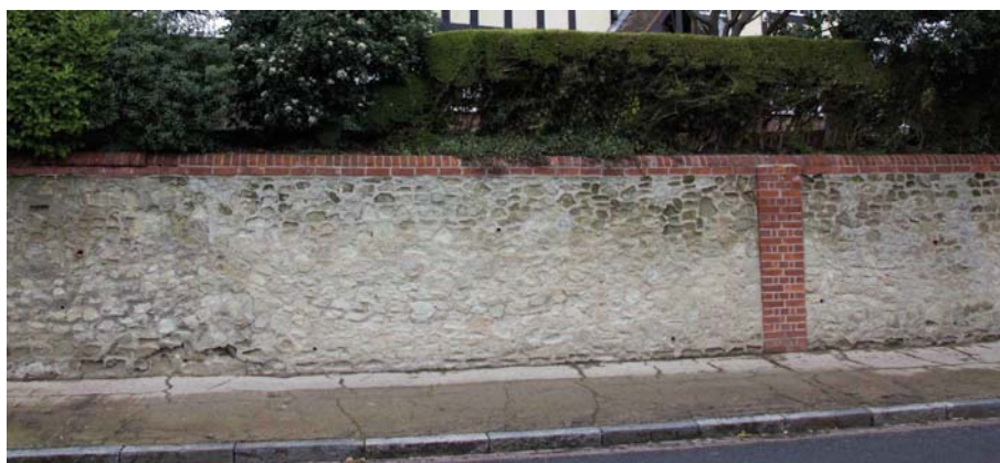
Picture 21 Example of original boundary walls.
