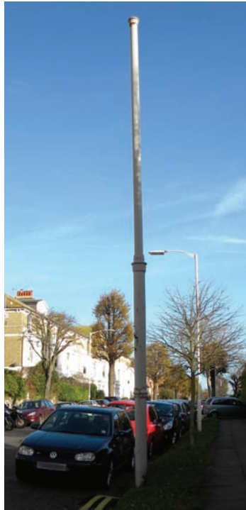
Picture 35 Vent pipe Enys Road
