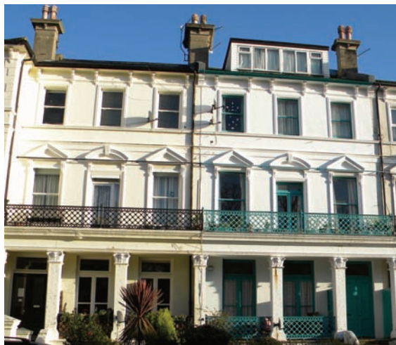
Picture 42 Prominent dormer to terrace, Upperton Gardens.
