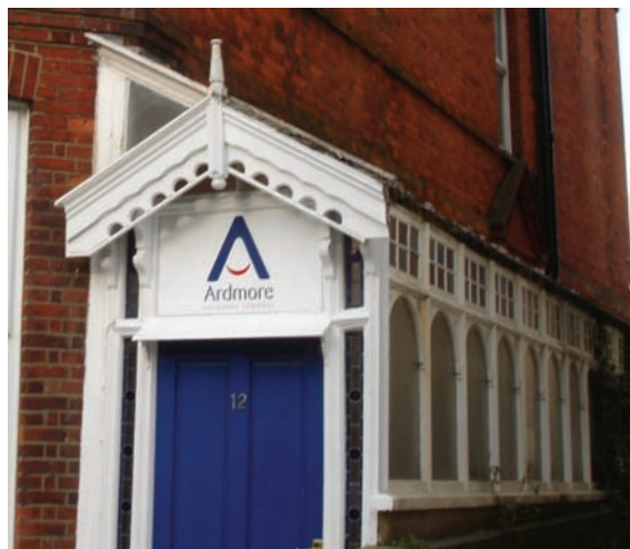
Picture 24 Porch to no. 12 Eversfield Road.
