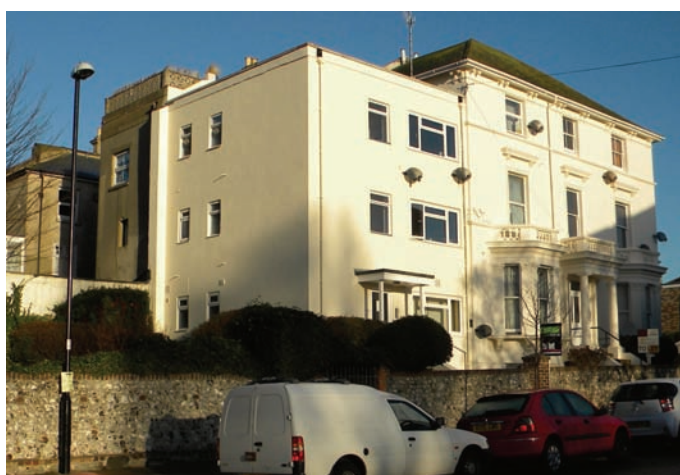
Picture 45 Dominant rear extension Upperton Gardens.
