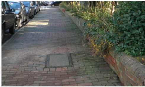
Picture 46 Traditional brick paving Hartfield Road.
