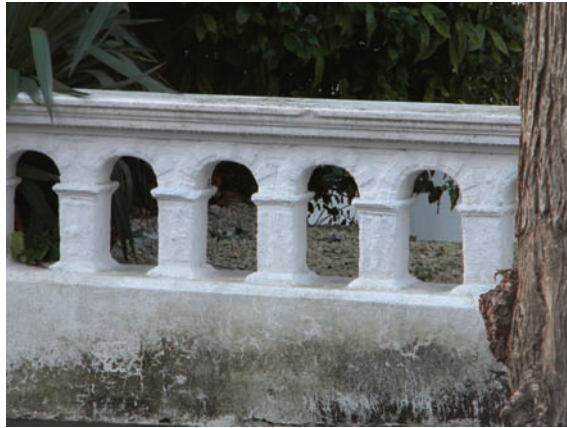
Picture 25 Boundary wall to locally listed terrace St Anne's Road.
