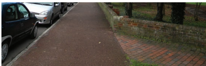
Picture 38 Footway paving Hartfield Road.
