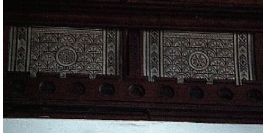
Picture 42 Ceiling panels to Christ Church nave.
