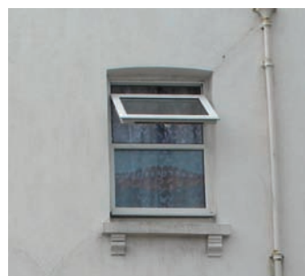
Picture 55 Replacement UPVC window.
