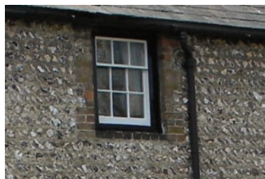
Picture 51 Original timber sash window to Church Cottage.
