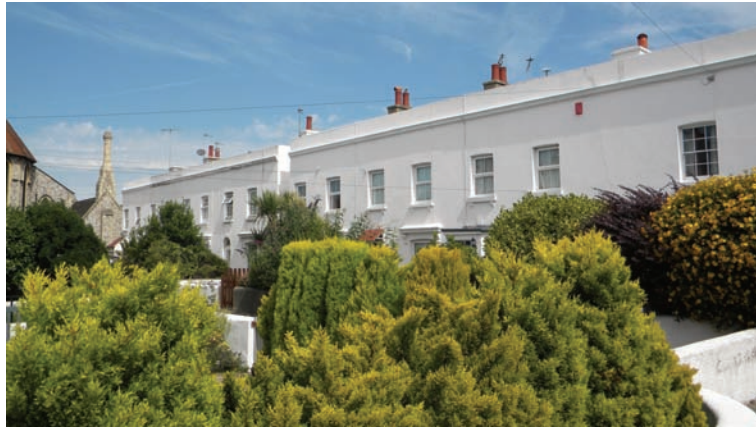
Picture 20 Chimneystacks to Warrior Square, nos. 1-8.
