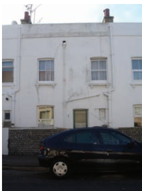
Picture 26 No. 6, rear elevation (Hanover Road).
