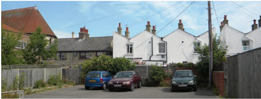
Picture 18 View of the rear elevations from St James Road.
