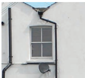
Picture 52 Original timber sash window, Warrior Square.
