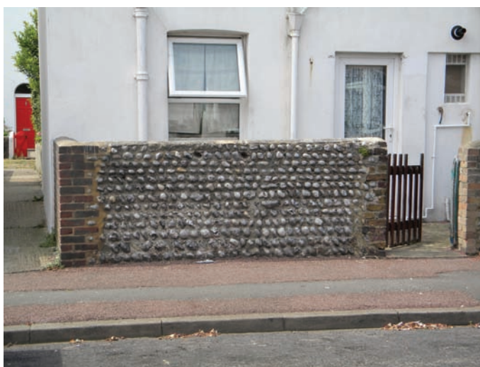
Picture 46 Flint wall, Hanover Road.
