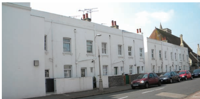
Picture 5 View from Hanover Road towards Seaside.
