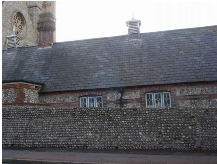
Picture 59 Flint walls to Hanover Road.
