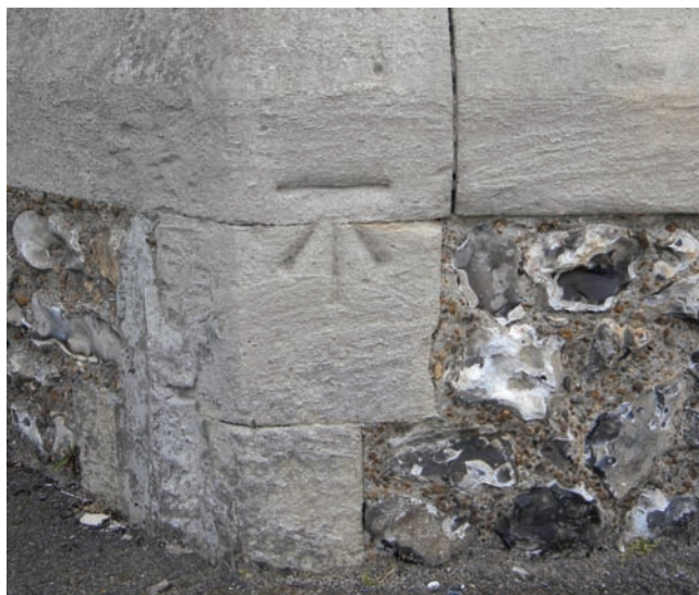
Picture 40 Benchmark to tower plinth.
