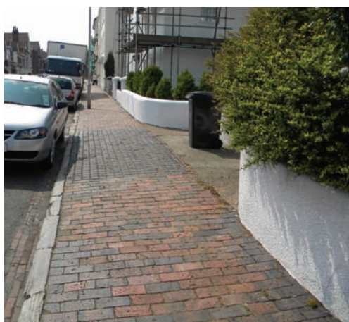
Picture 47 Pavoids and Staffordshire blue bricks to Latimer Road.
