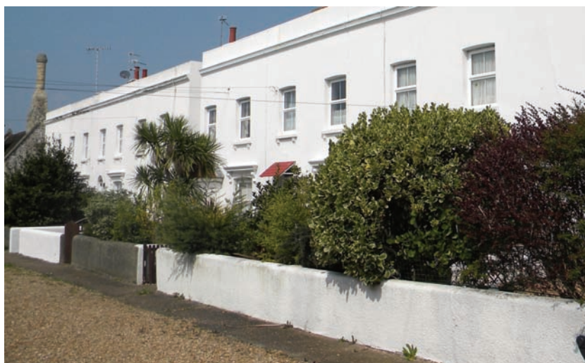
Picture 58 Warrior Square, boundary walls.
