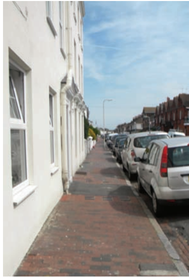
Picture 60 View of footway, Latimer Road.
