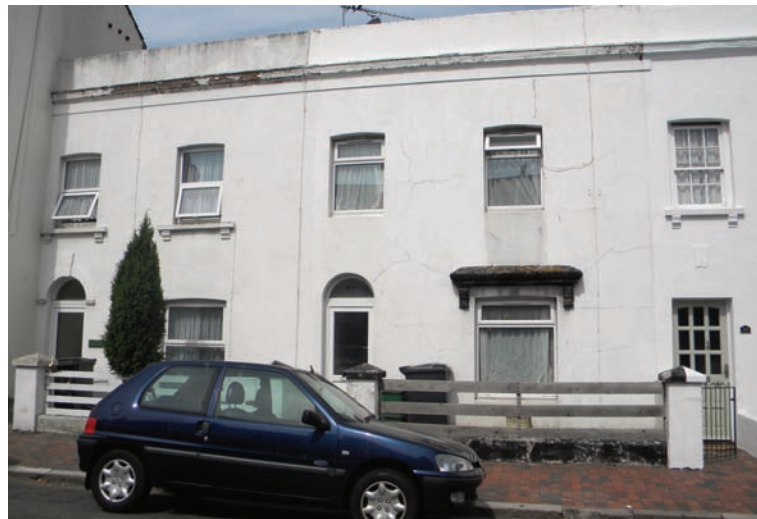
Picture 57 Latimer Road, all original windows & doors replaced & fanlight infilled.
