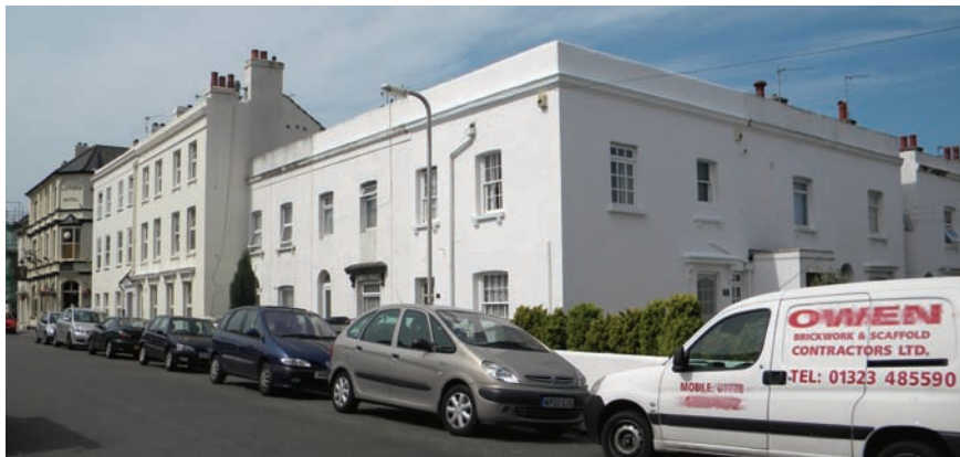
Picture 35 View of nos. 31, 33, 35, 37 and 39, Latimer Road.
