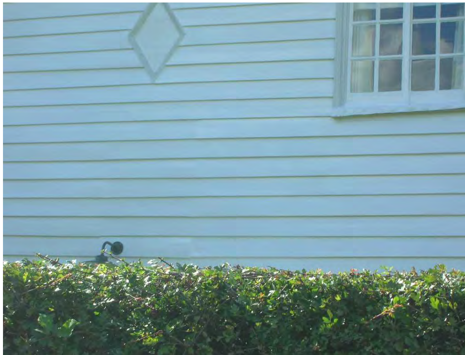
White Lodge, Church Lane, detail of white painted weatherboarding and timber casement window
