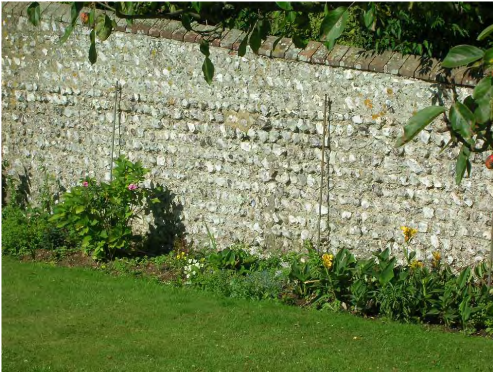
The Lodge, Church Road example of a field flint wall located on a side boundary
