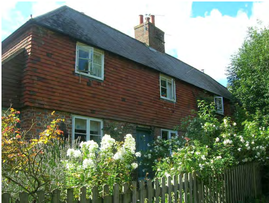
Beeches Cottages, Church Road, with red clay hanging tiles on the first floor
