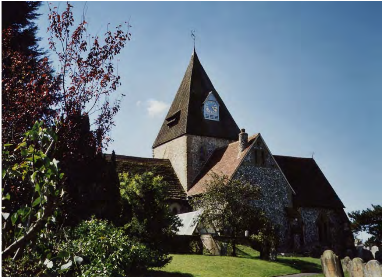
The church is roofed with clay tile and Horsham stone slabs
