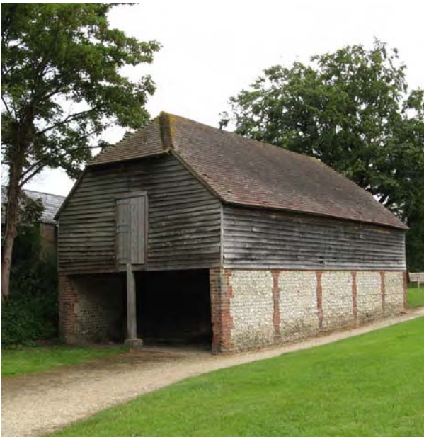
Eighteenth century barn beside the village green
