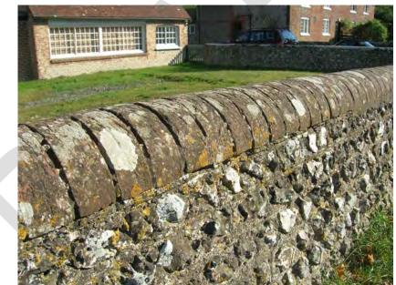
Wall constructed of field flints with contrasting half round red brick coping
