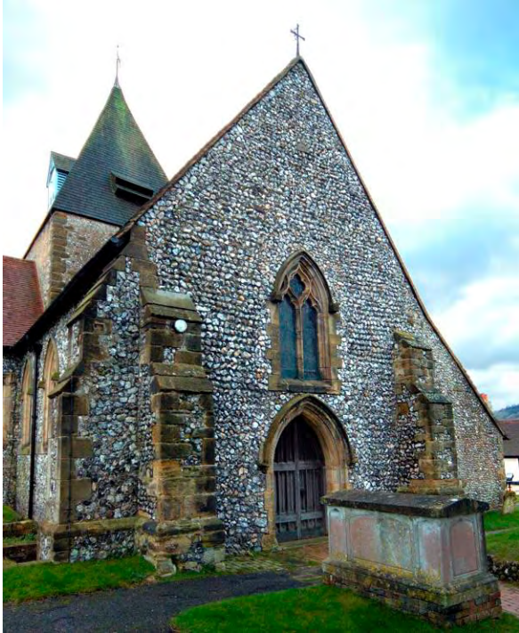
Fig. 10. St Margaret's church: west wall of nave.
