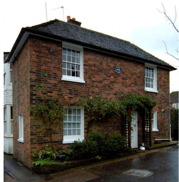
Fig. 17. Ford Cottage, 42 East End Lane (c.1812).
