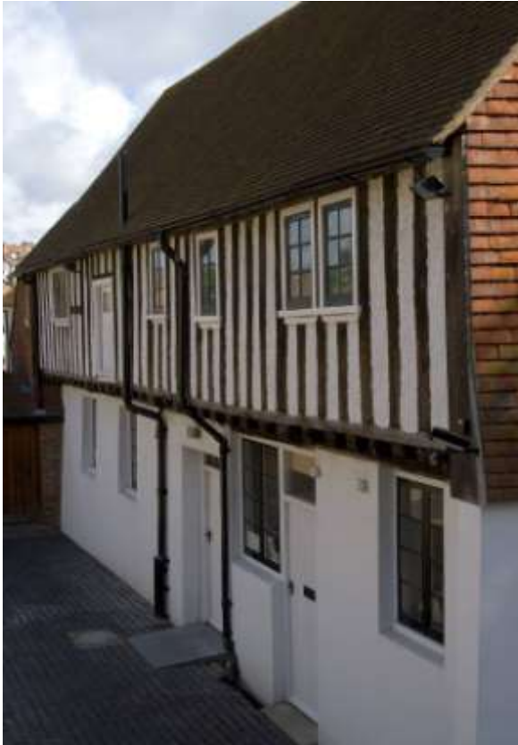
Fig. 26. Old Parsonage Barn: west elevation.
