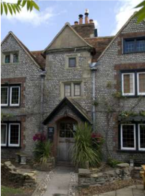
Fig. 29. The Counting House, Moatcroft Road.
