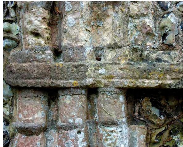
Fig. 16. St John-sub-Castro: detail of re-sited 11 th -century doorway (see also Fig. 3).
