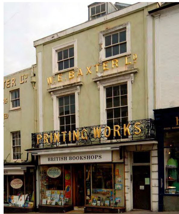
Fig. 38. 34 High Street (School Hill): early 19 th -century stucco refacing of 16 th -century timber-framed townhouse.
