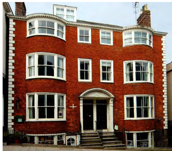
Fig. 33. 199 and 200 High Street (School Hill): late 18 th -century mathematical tiles and wooden quoins.
