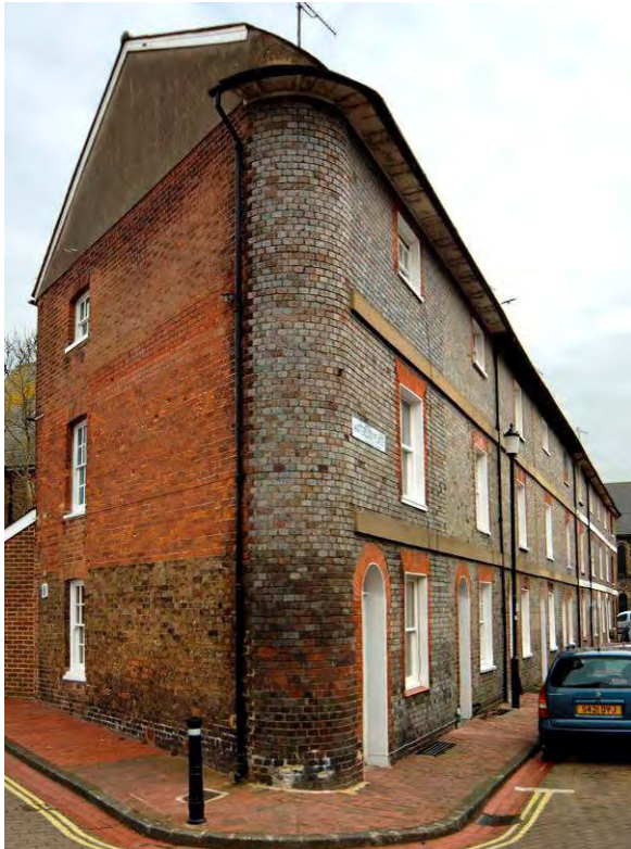
Fig. 37. Waterloo Place: early 19 th -century terrace with brick façade to flint-rubble walling.
