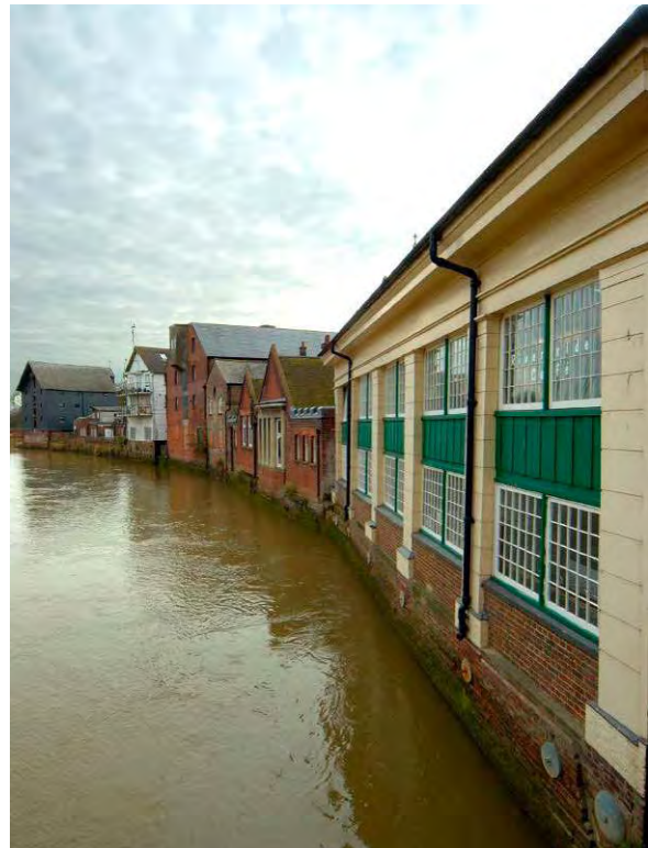
Fig. 40. Warehouses on the west side of the River Ouse, south of Lewes Bridge, from Riverside (foreground) to Stricklands Warehouse.
