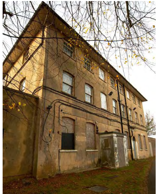
Fig. 13. Newhaven Union workhouse, Church Hill (1835).
