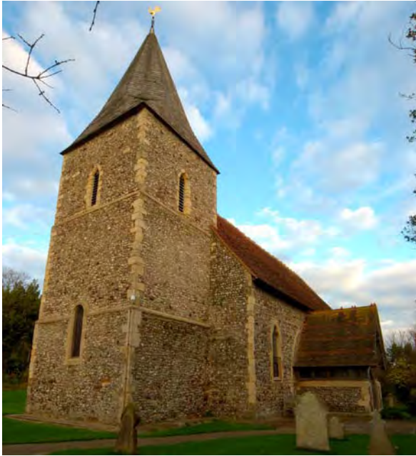
Fig. 7. St Peter's church, East Blatchington: view from SW.
