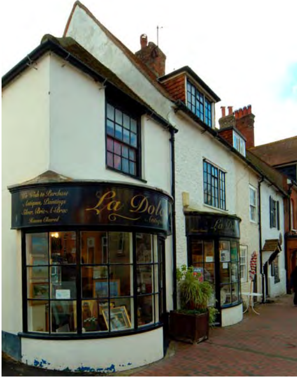
Fig. 11. 44-50 High Street. Behind the early 19 th -century No. 50 (foreground) is the gable of a timber-framed 17 th -century house, re-fronted with cobbles c.1800.
