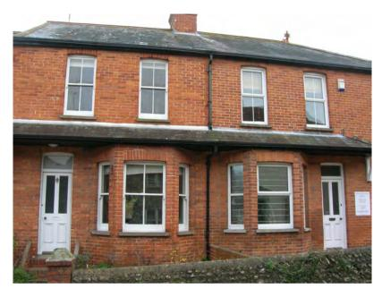
Above: The timber sash windows in this Victorian terrace are retained in the property on the left but have been replaced with uPVC in the property on the right. uPVC cannot accurately replicate the quality or character of the original sash windows.
