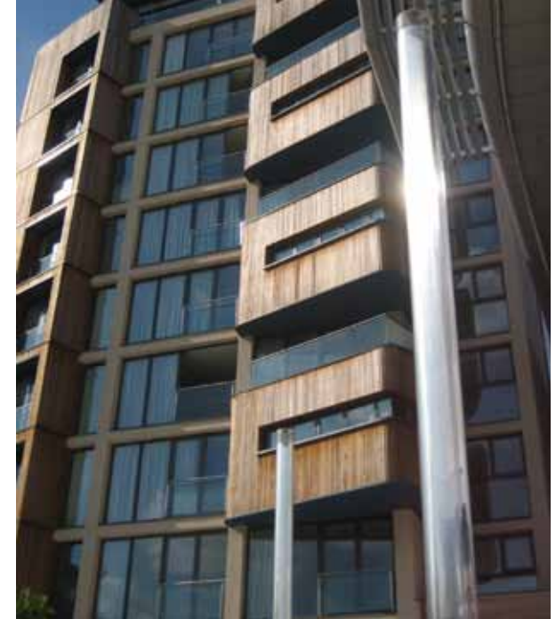
Apartment building provides a distinctive built form
