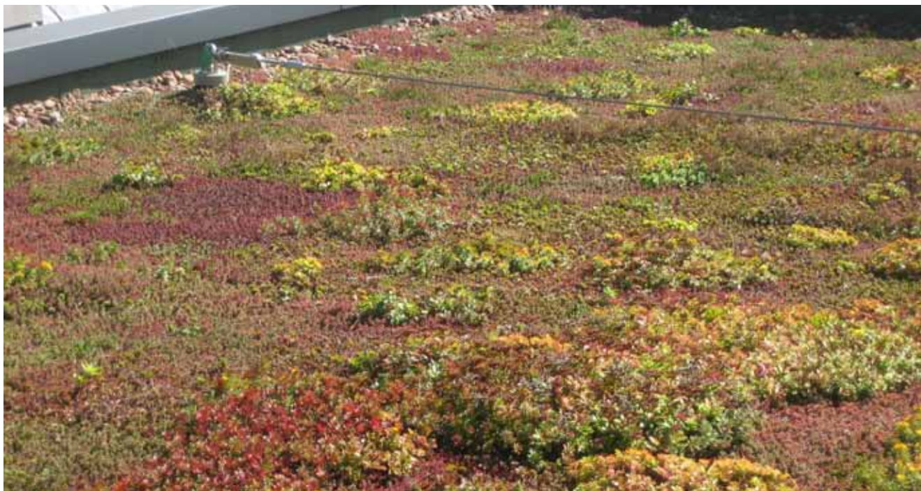
Example of a green roof
