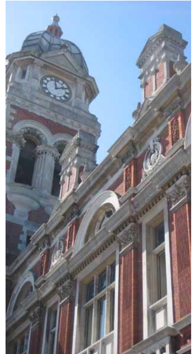
Town Hall - a distinctive landmark
